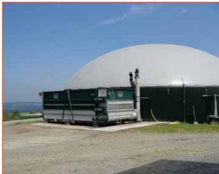
Dry feeding system with 38m 2 developed for manure and grass
