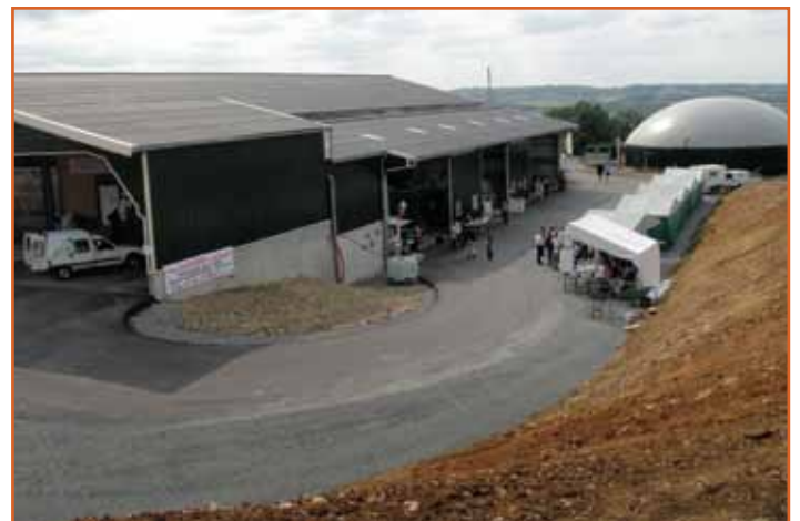
Grand opening and commissioning of the agricultural biogas plant
